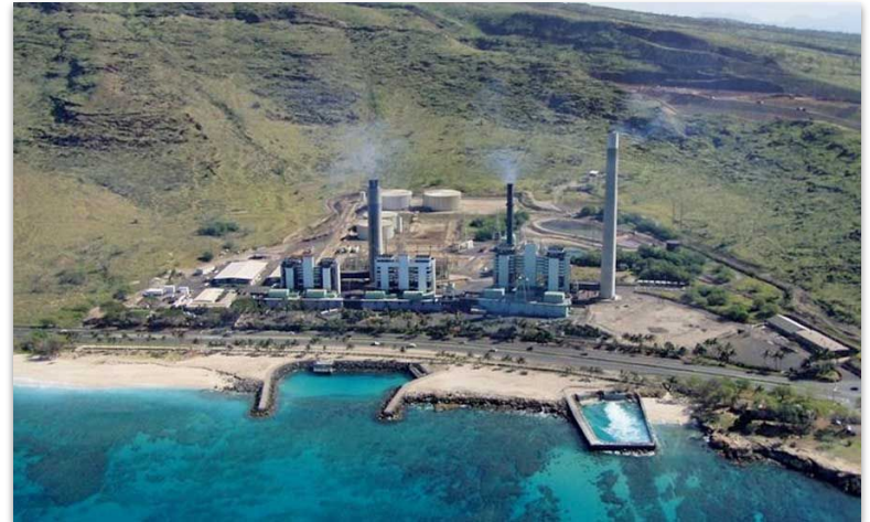
Kahe Power Plant
